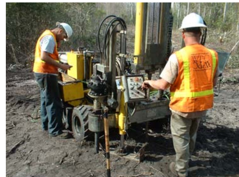
WPC CPT rig and operators
