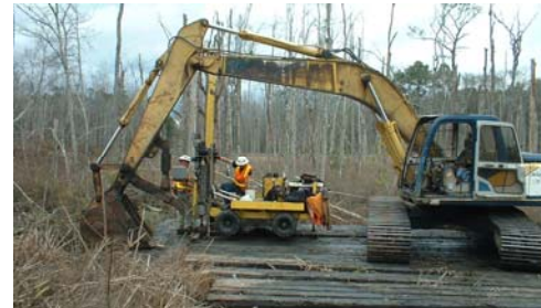
CPT working from timber platform
