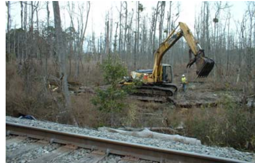
View of work from existing track
