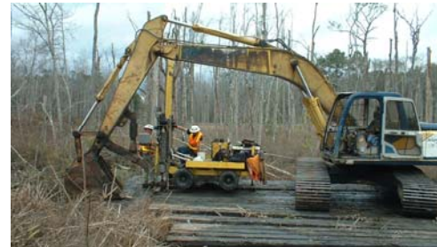
CPT working from timber platform
