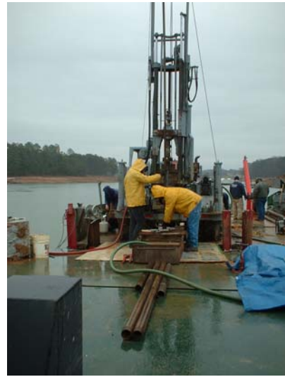
Drilling from barge in poor weather
