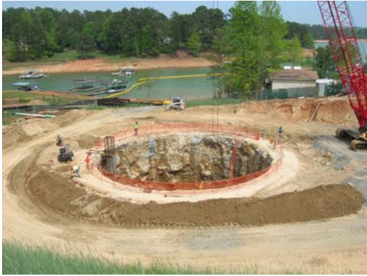
Excavation for project wet well
